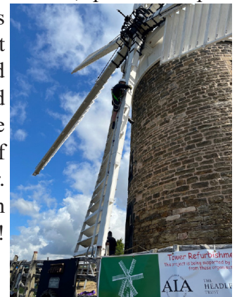
Lime mortar part completed.
