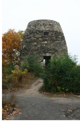
The empty mill tower in October 2009 (photo Ton Meesters)
