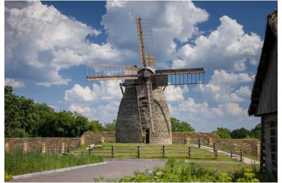
The restored mill in 2024 (photo Andrey Avdeenko)
