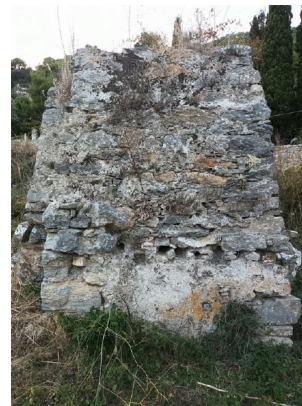
Fig. 6. On the eastern side of the drop tower, the holes for supporting the wooden beams of the watermill roof are visible (photo by I. Papaeftychiou).
