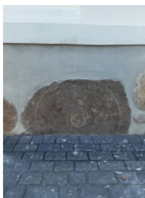
4. Example of an unfinished millstone set into the wall base of a church in Mazovia (photo by D. Brykała).
