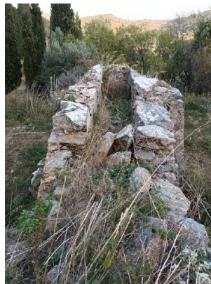
Fig. 5. The square cross-section of the drop tower, as seen from the mill race (photo by I. Papaeftychiou).
