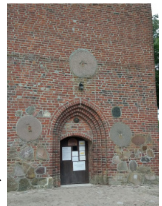
1. Three medieval millstones embedded around the main portal of the Gothic church in Pomerania (photo by D. Brykała).
