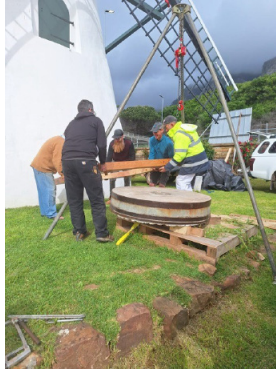
Testing the curb over the up-turned bedstone.
