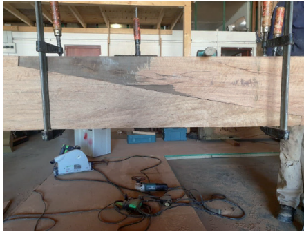
One shear has its outriggers fitted. The four bolt holes for the clamps at the scarf can be seen. The second shear is in the foreground. The outriggers will be cut to length when we have worked out how long they must be, and finished with fancy "ogees".
