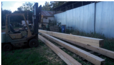
Selecting the straightest pair of spruce beams for the long stretcher.
