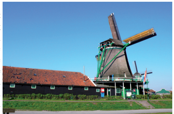
Oil mill De Zoeker, Zaandam, The Netherlands. Photo Leo van der Drift, April 2010.
