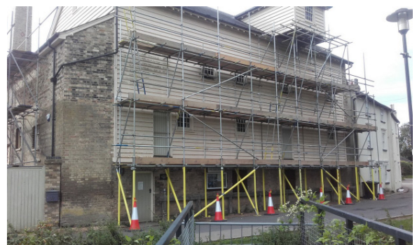
Fig. 3. Stotfold Watermill in scaffolding.
