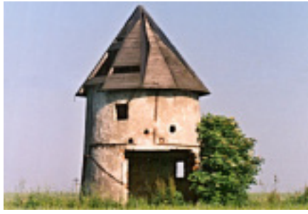
1. Spálov, before reconstruction, 2004, photo by J. Doubek.
