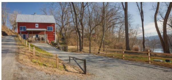
Our newly repainted and reroofed, cupola-sporting mill. All photos by Dan Chung Photography
