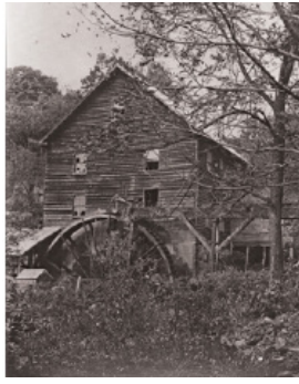
Figure 3. Locke's Mill c. 1920
