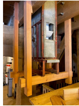
Organic grain elevator boot to receive bulk grain and convey to third floor grain bins.
