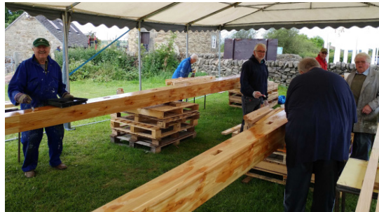
All the new timber was given a coat of sealant.
