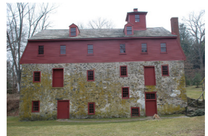
Newlin Grist Mill, outside view.
