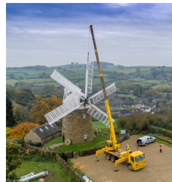
The first of the new sails is lowered into position.
