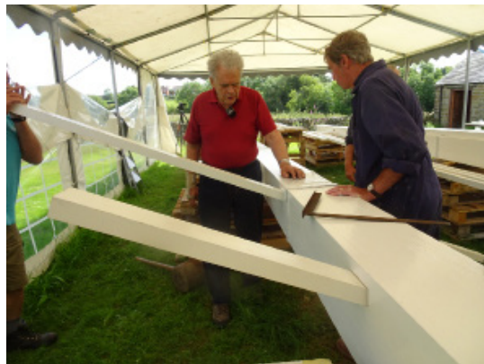
The first sail bars are cautiously fitted.
