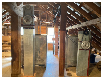
Third floor elevator heads. Water powered hopper, bottom grain bins in background.
