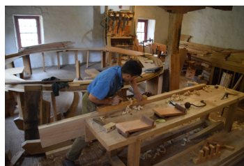
Squaring planks for flume sheathing.
