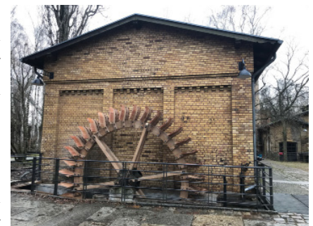
The Technical Museum watermill after fitting the new wooden waterwheel.
