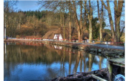
1. The mill dam or weir at Lille Mølle near Nyborg on Fyn. Earlier there were some problems with the spillway gate, requiring some repairs to the sluices (see bottom right in the picture). Photo: Per Gliese.
