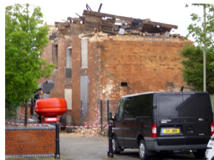
Photograph 10 taken 3rd August 2017: The bin divisions in the loft are revealed.
