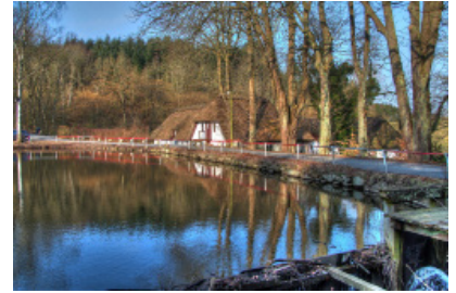
1. The mill dam or weir at Lille Mølle near Nyborg on Fyn. Earlier there were some problems with the spillway gate, requiring some repairs to the sluices (see bottom right in the picture). Photo: Per Gliese.
