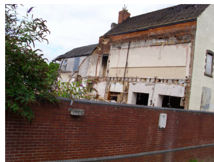
Photograph 6 taken 31st July 2017: The original rear of the mill exposed.
