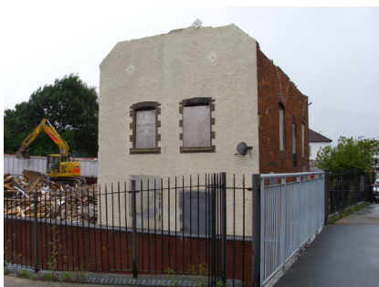
Photograph 9 taken 2nd August 2017: From the west end, over the footbridge.
