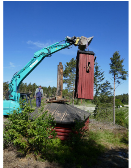
Lifting the buck of Söderlångvik estate windmill (photo by Kirsti Horn).
