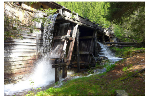
The Wegelate Saw Mill at Innervillgraten, Austria, is one of the mills featured (photograph by Leo van der Drift)
