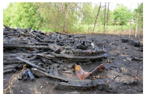
The remains of Keminmaa smock mill (photos by Matti Viljakainen).
