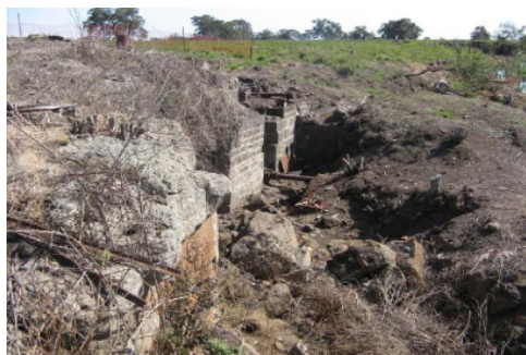
Fig. 4. Thomas Mill on the Plenty River showing the wheel pit and remaining gearing (photo Gary Vines)
