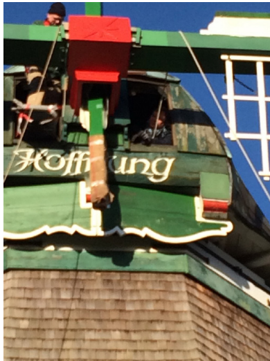
Replacing the outer sail stock at Munkbrarup Windmill.
