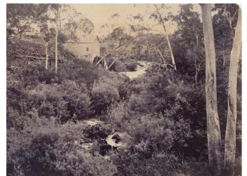
Fig. 3. Carome Mill in the 1850s (State Library Victoria).
