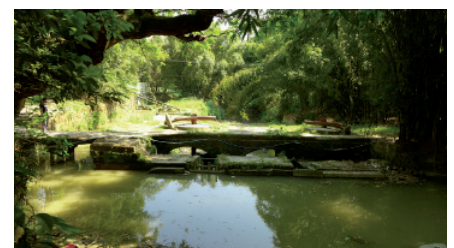
The bridge seen from upstream
