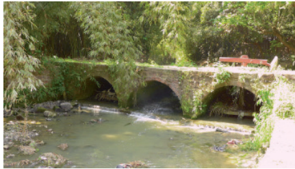
The bridge seen from downstream
