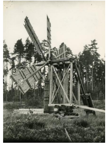
Skeleton mill (shingle mill) at Korteniemi Farm, Letku near Tammela, Kanta-Häme region (coll. The Mills Archive, Reading, UK).
