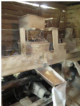
20 Wheelpit, hopper and stones
