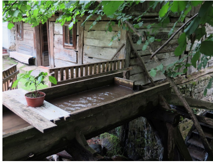
12 The flume bringing water to the mill
