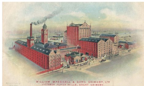
Victoria Flour Mills, Great Grimsby, Lincolnshire, a roller mill plant.
