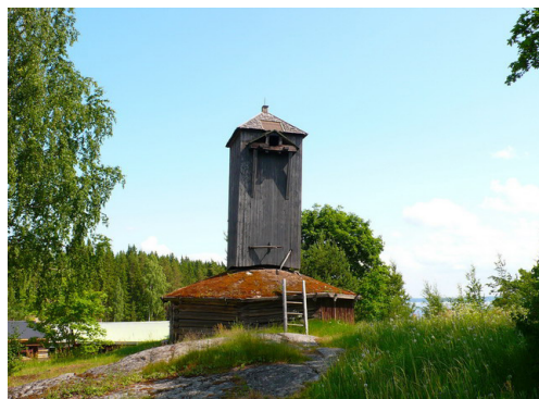
Hollow post mill at Vikelä farm, Ylöjärvi (Pirkanmaa). Picture 2011, but since restored (Photo Leo van der Drift).
