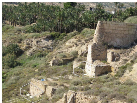
Figure 2 Remains of Rambla mills. Right: the penstock (pressure shaft) of the upper mill. The contours of the former mill houses, of the wheels and the penstock of the lower mill are sketched.
