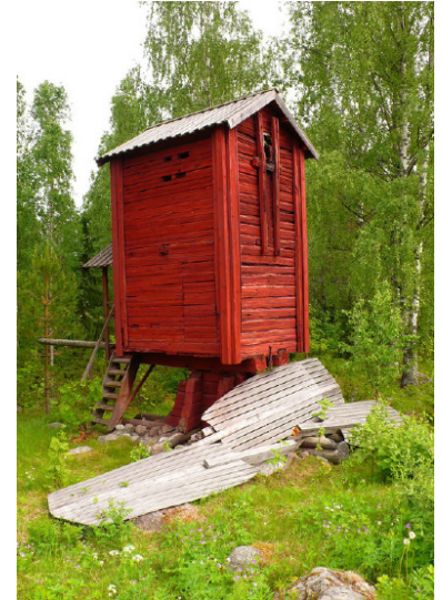
Post mill “Saaninveden mylly”, at Ilsojoki, Pihtipudas municipality (Keski Suomi), having lost its sails (Photo Leo van der Drift, 2011).
