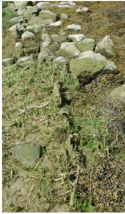
Pond-side sheathing, Paine Mill, Woolwich ME
