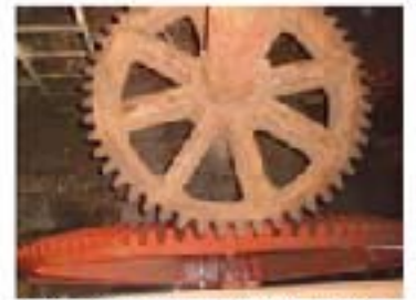
Looking down on the new pit wheel in situ.
