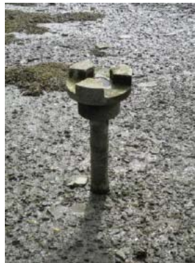
Probably a 19th century iron turbine in the mud at the Friend tidal mill site in Beverly. [Photos: Earl Taylor]
