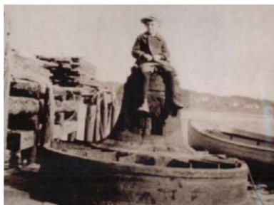
Probably a 19th century iron turbine in the mud at the Friend tidal mill site in Beverly. [Photos: Earl Taylor]
