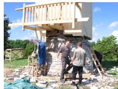
Village men repairing the stone foundation.
