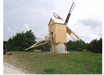
The windmill after restoration.
