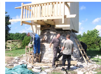
Village men repairing the stone foundation.
