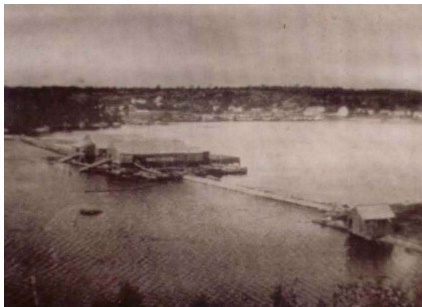
Morse Dam– Winnegance in background (Photo: MMM)
