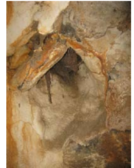
The chimney above the hearth
