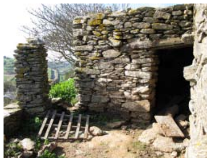
The porch and the kitchen entrance with the oven
