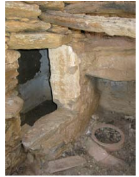
The flour storage bin (left) inside the mill basement
