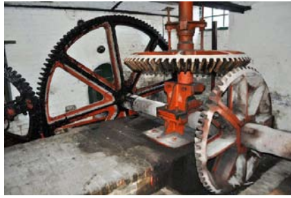
The gearing system for one grinding pan
