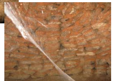
The oven inside. Note the red ceramic clay between the stones
