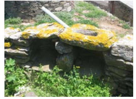
Ledges underneath the trough. Ledges of all shapes are found all over the building and in the stone fence for various purposes.
