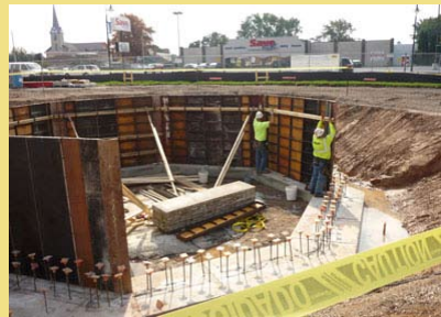
Windmill foundation under construction
