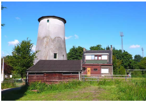
The Babbersmolen awaiting completion.
