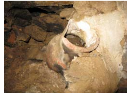
Small clay pitcher built in the wall next to the hearth used for cutlery
