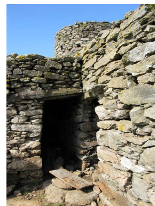
The kitchen entrance (left) and the house entrance (right)
