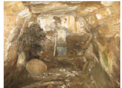
Inside the house (western side). On the left corner the hearth, in the middle the cupboard, below one of the stone beds. At the hearth they were making cheese and heating water to knead. Notice the roof stone beams. Notice the leaning walls inwards
