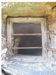
The only window on the eastern side
