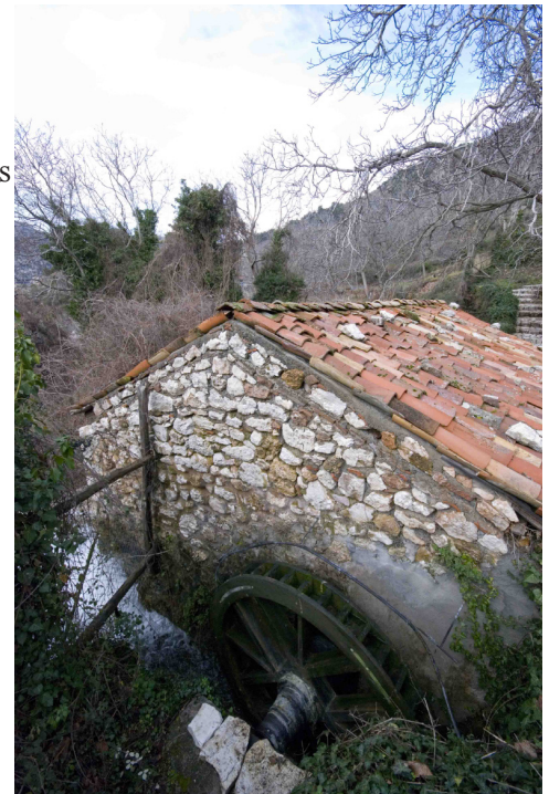
The upright wheel of the gunpowder mill
