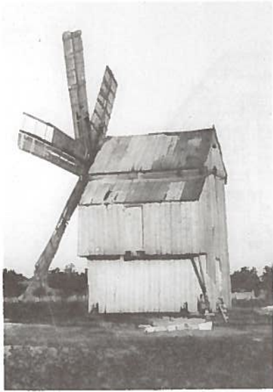
Fig. 34.29 R-50 010-Sabangia Mill, Județul Tulcea. UTMn 35/647/4987. Post mill with two stories and two pairs of stones - of the same type as R-50 003, pictured to left and right.
