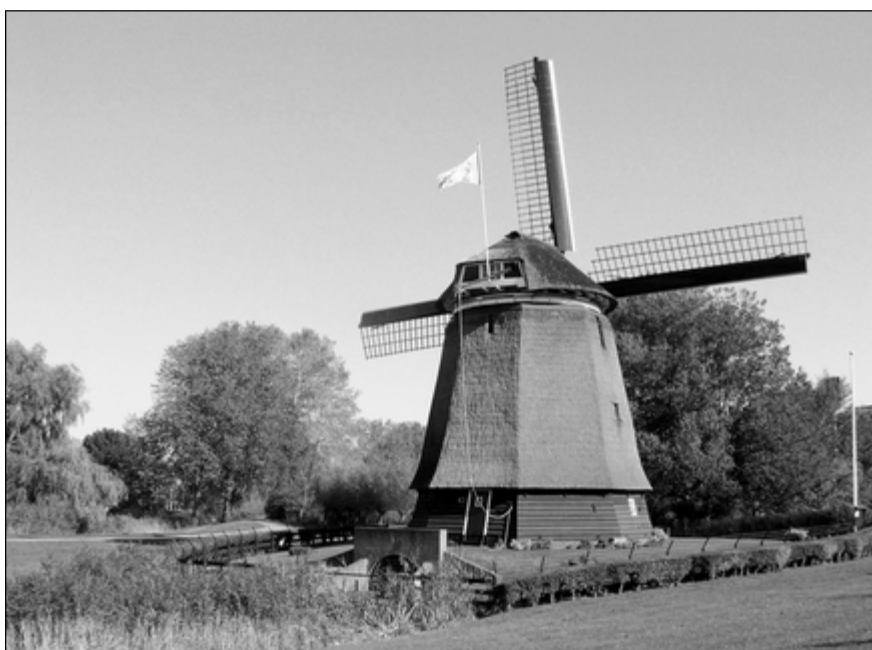
Fig. 4. Drainage mill De Geestmolen at Alkmaar, built c.1560, is among the oldest preserved octagonal smock mills in The Netherlands. Photograph by H. Kaptein.
