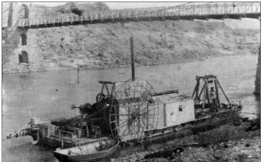
Fig. 4. Victoria dredge post-1897 in derelict condition near the old Alexandra bridge across the Clutha River, retaining only one paddle wheel frame.
