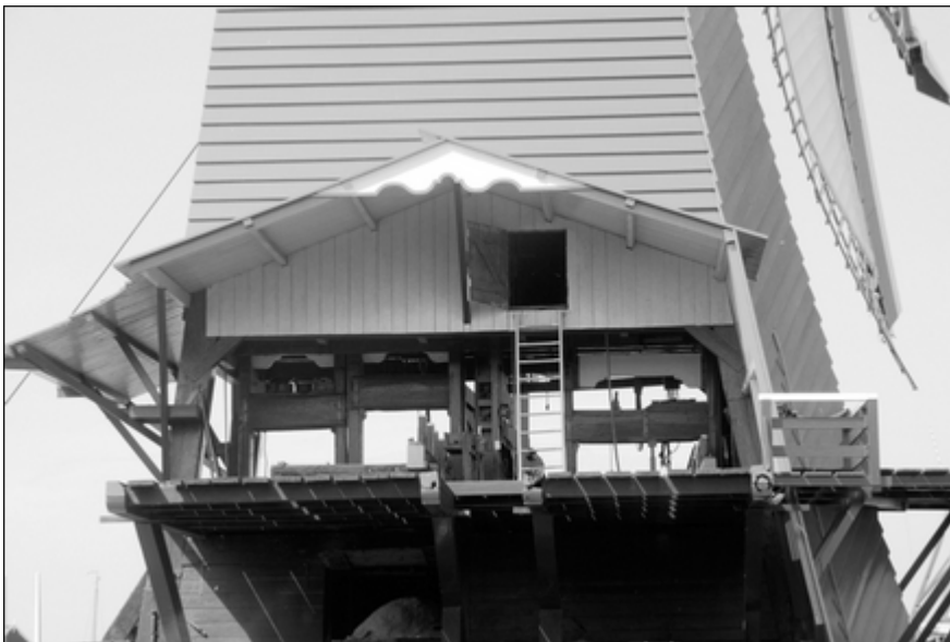
Fig. 5. Cornelis Cornelisz van Uitgeest, the inventor of the wind-driven saw mill, used a crank shaft so that the saw frames perform a reciprocating movement. Paltrock mill De Gekroonde Poelenburg at the Zaanse Schans.
