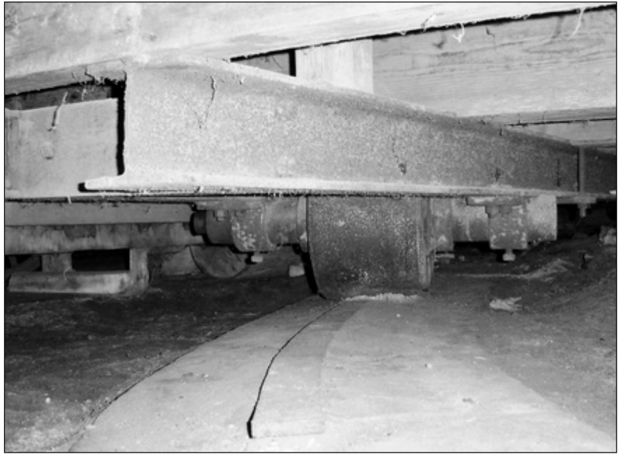
Fig. 6. One of the large wheels under the extended mill running on the iron rail on top of the concrete circle.
