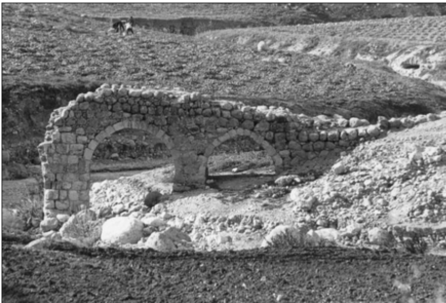
Fig. 14. The remains of the aqueduct carrying the leat to the sugar mill at Krayma
