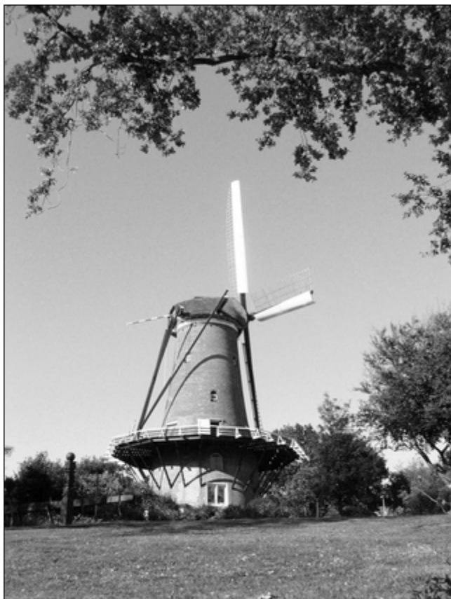
Fig. 1. In almost every town, one or more windmills with reefing stages can still be found that in most cases were used for grinding grain. Photograph by H. Kaptein.
